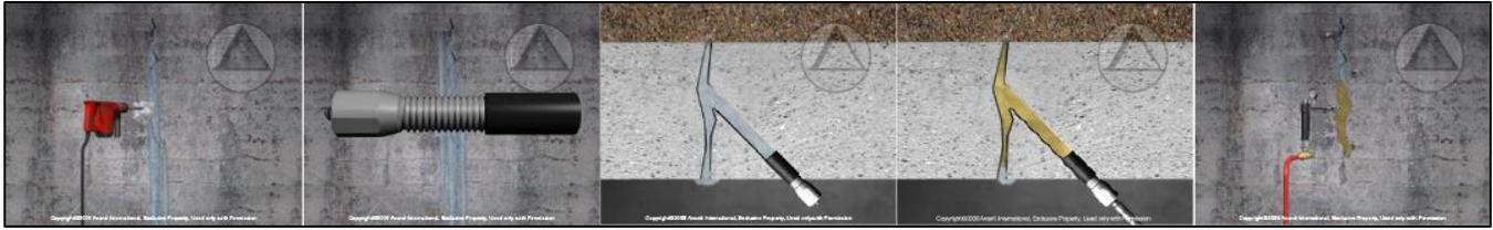
**Photo 1.** Steps of the Crack Injection Process
