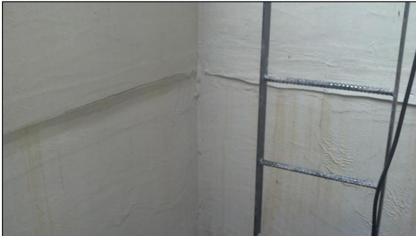
**Photo 2.** Indication of water intrusion and rundown in vault.
