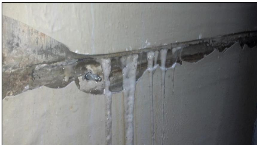
**Photo 3.** The joint was injected with a flexible hydrophobic grout.
