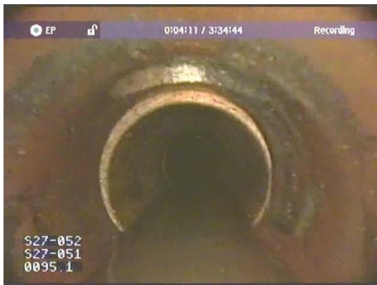
Figure 6. Sewer main & lateral pre dye flooding
