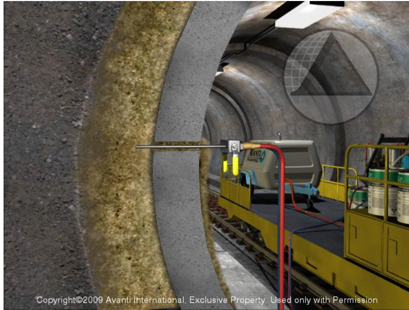
Figure 3. Chemical grout permeating the soil to create an impermeable grout curtain
