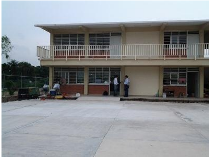
Figure 5. Photograph of the west end of the school building near the retaining wall
