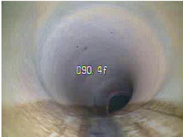
Figure 1. Immediately After Installation Inspection
