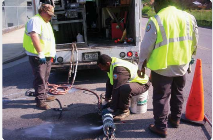
The City of Chattanooga, TN, has been a city in the forefront of grouting over the last 20 years, using it to solve I/I issues.
