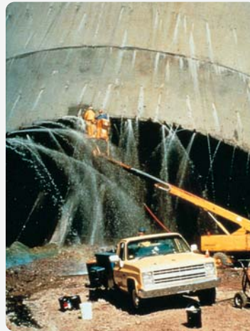
View of grouting and leak cessation.
