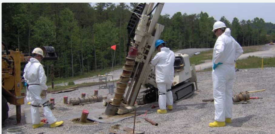
Collar pipe installation at ORNL trench.
