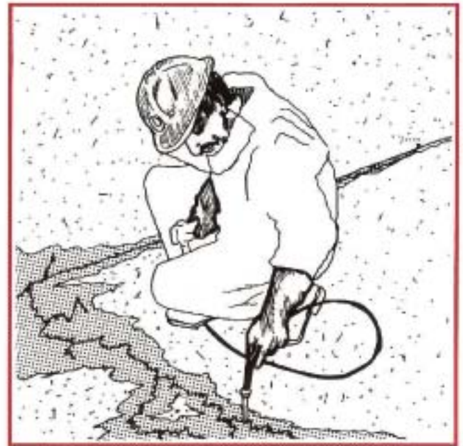
Injection of PUR grout into floor slab crack. Note disposable coveralls and protective equipment.
